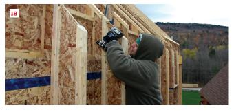
instead, we framed the wall straight across. But now that it was time to trim the wall to match the angle, we laid our rafter against it and scribed for the cut (10). Then we transferred the line to the outboard face of the wall and cut the scrap part off (through the sheathing) using a circular saw (11) and cut the studs using a recip saw. We pulled the little scrap piece off (12), framed in the gable, and then set our end rafter on the new plate (13).
